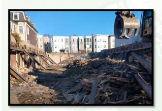
The majority of material derived was classified as C&D (Construction and Demolition) which was brought to Stoughton Recycling. Stoughton uses a state-of-theart mechanical process to recover wood from the waste stream, which is then sorted and sized into a specified bio-fuel for a regional wood-fuel-derived power plant.
