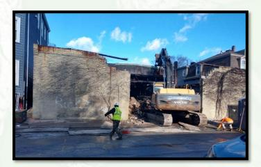
Using a combination of careful manual and mechanical methods, we separated structures from the perimeter walls to remain and lowered small sections of roof and truss to the ground. Sorting of all building components for recycling took place within the building footprint. The congested nature of this residential area did not allow for on-street truck loading, so the crew created access for haul trucks to the footprint by removing building bays in succession.
